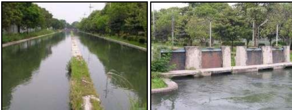
Figure 3: raw water intake (left) and flood gates (rights) at the Ngagel water treatment plant.
